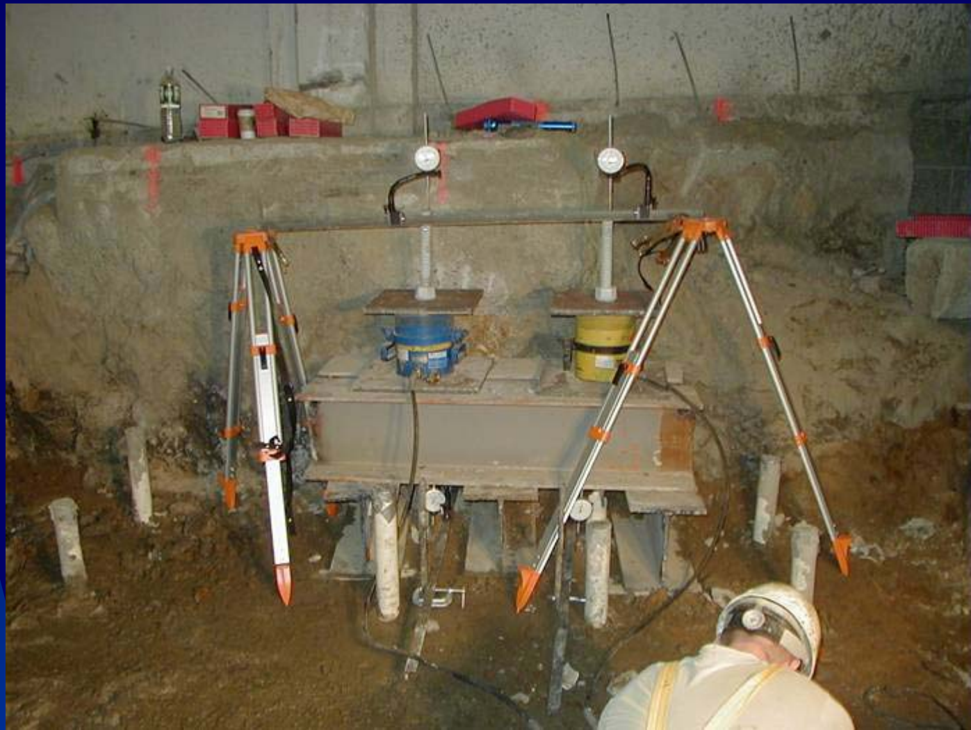
Typical tension test set up for a pile group
